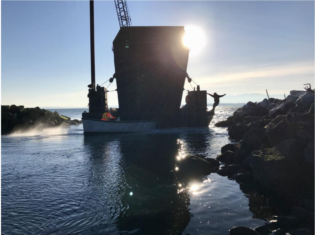
The piling barge entering the jetty.
